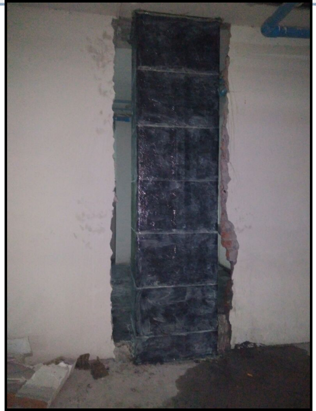
Build Wrap UTS 300, apply on Column
